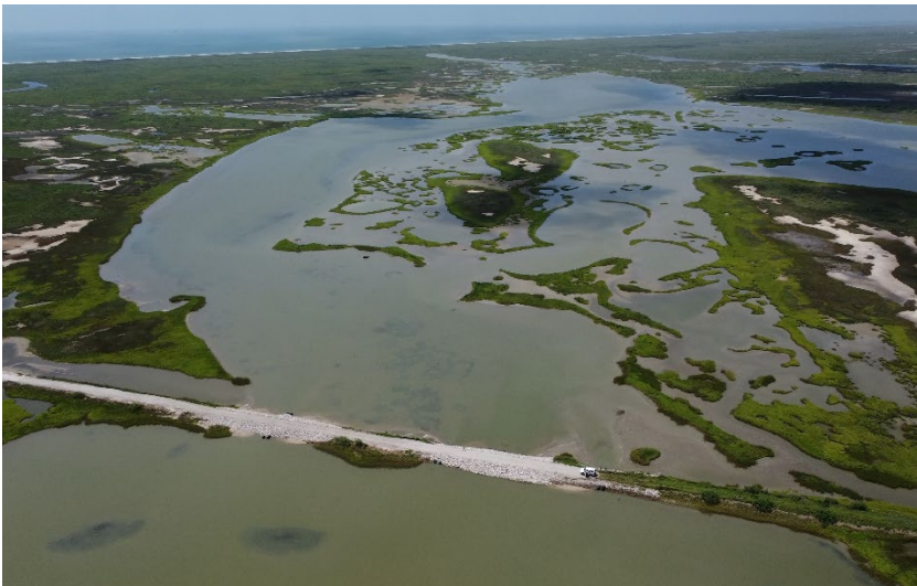
Completed Matagorda West Marsh Levee Restoration
