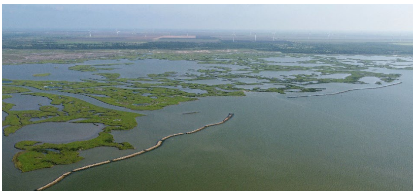
3,600 ft breakwater structure protecting the Nueces Delta Shoreline.
