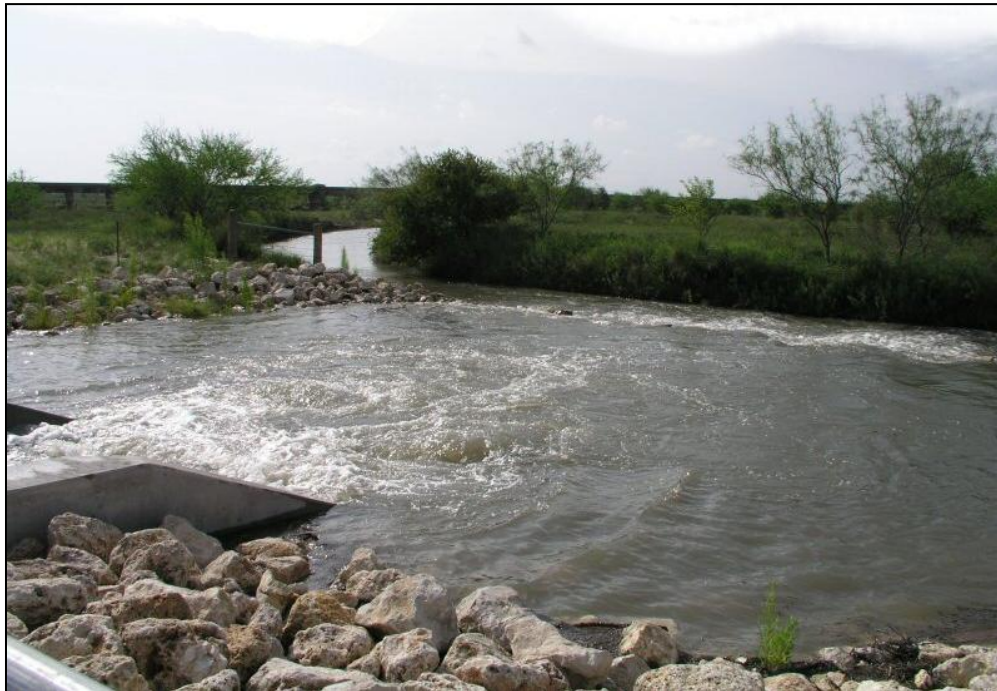
Figure 2-5. Rincon Pipeline outfall
