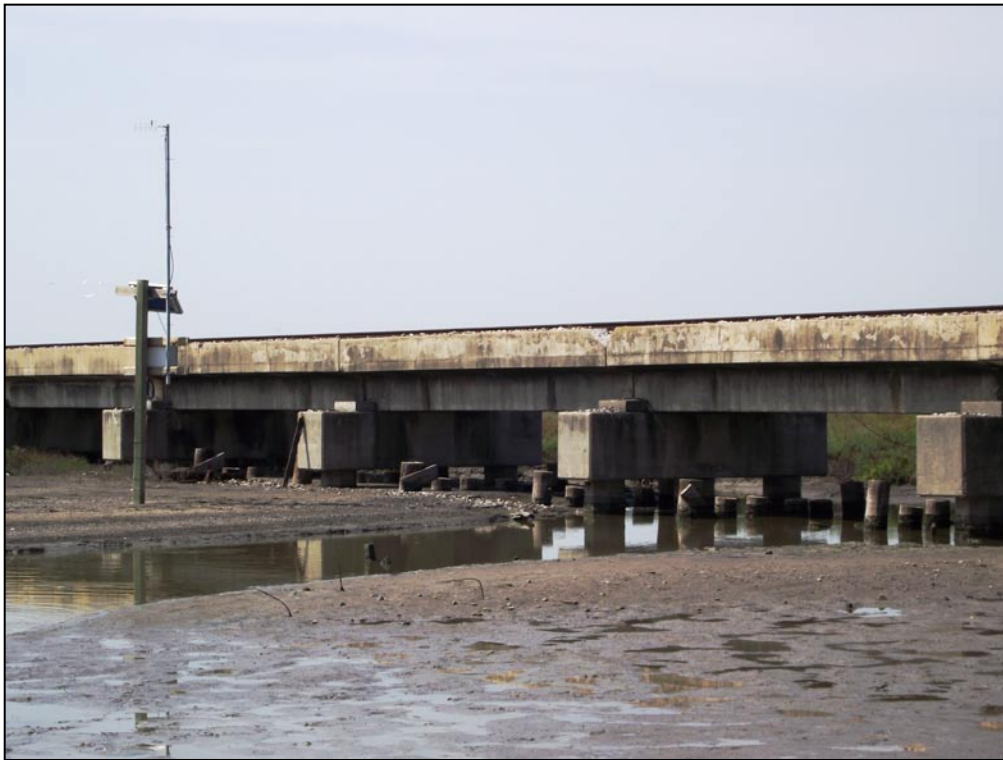
Figure 4. NUDE02 at the railroad crossing. The data sonde is under the railroad in the deepest part of the channel.
