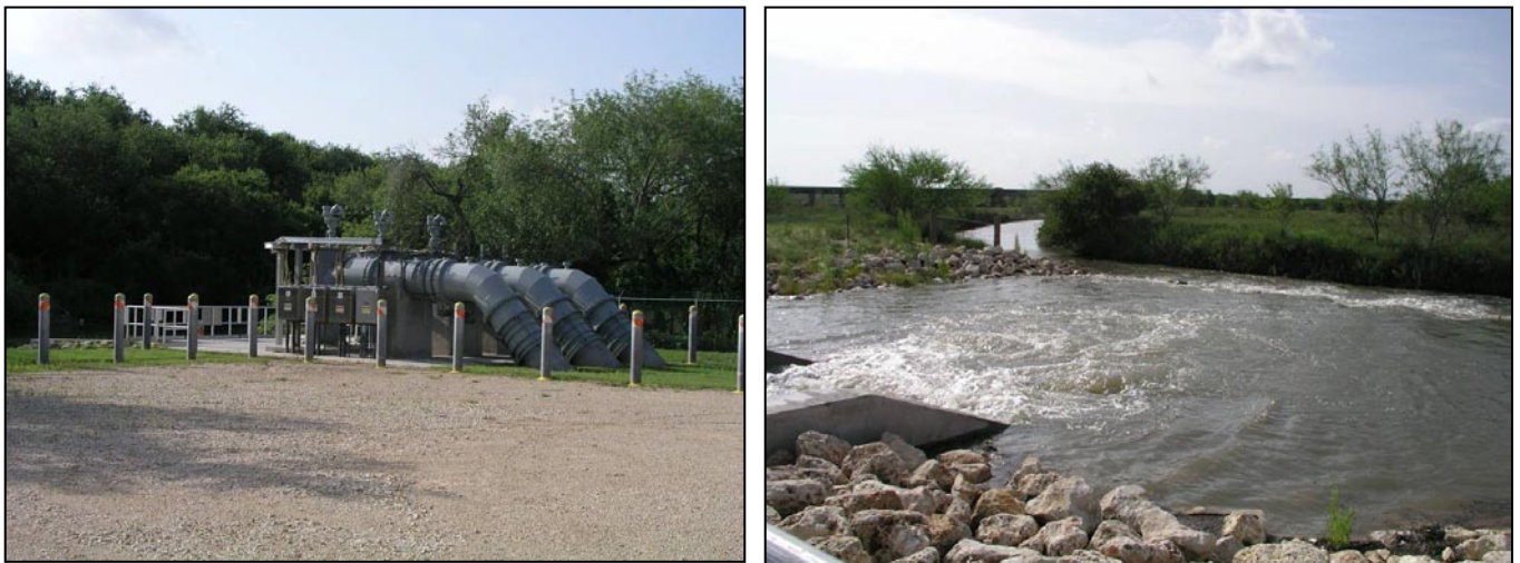
Figure 7. The left image is a picture of the pipeline intake pumps along the Nueces River. The right image shows the pipeline outfall along the Rincon Bayou in the Nueces Delta.
